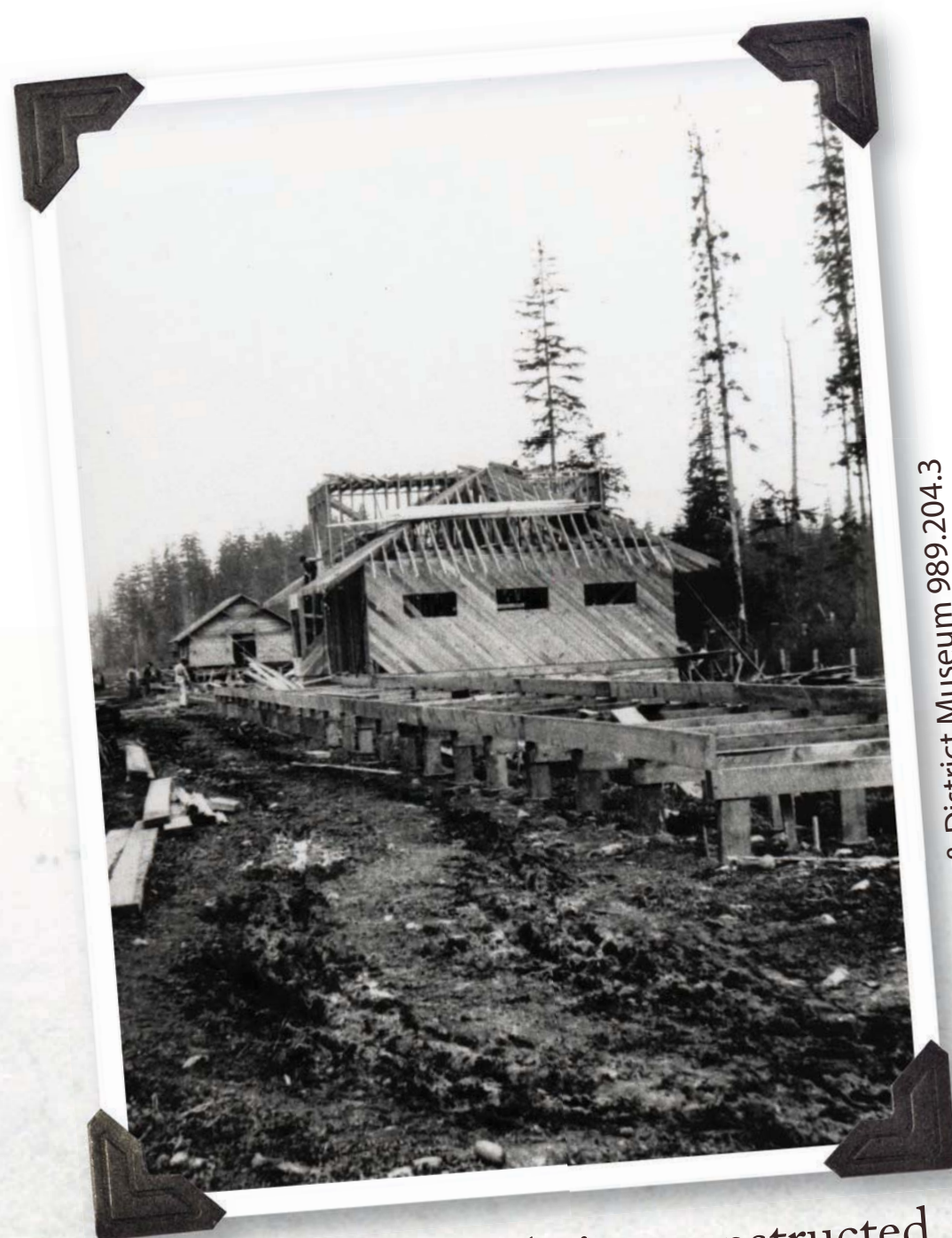
E & N Station being constructed
