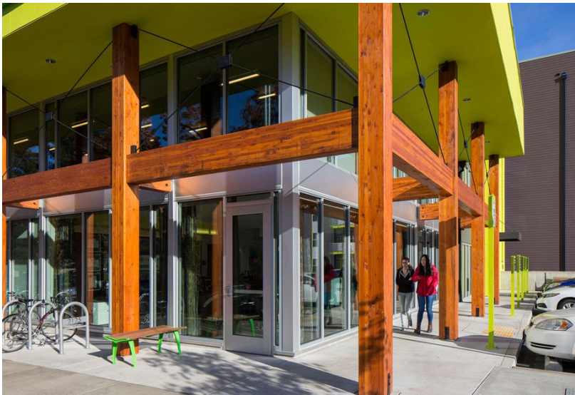
Example of using exposed mass timber structural elements as part of an emerging west coast character (guideline 23). Also includes pedestrian and cycling supportive features such as private sidewalks along the length of the building entry (guideline 56); weather protection (guideline 58); and seating and bike parking (guideline 31).
