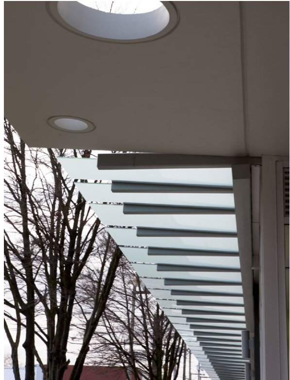
Example of a continuous weather protection option, such as along exterior building walls directly adjacent to pedestrian networks and areas (guideline 58).
