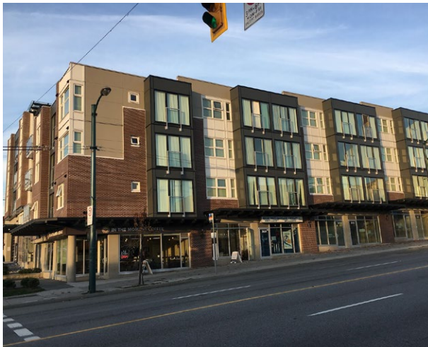
Example of articulated building frontages that are visually separated into smaller distinctive units, at both the ground and upper floors (guideline 15).
