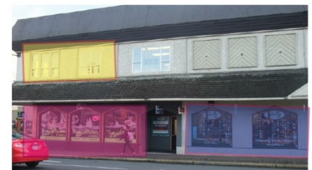
Each of the coloured boxes represents building face area for a different business premise
