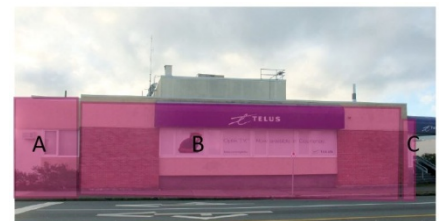
Together, A, B and C make up the building face area for this single tenant building
