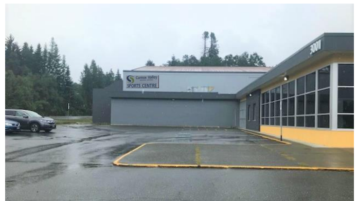
Figure 4: West Building Face (Source: Staff Site Visit August 1, 2019)
