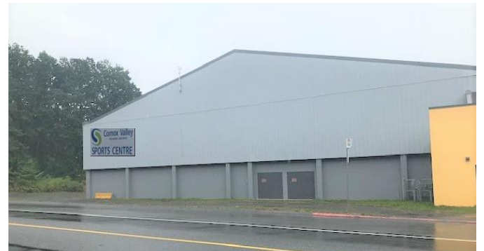
Figure 3: North Building Face (Source: Staff Site Visit August 1, 2019)
