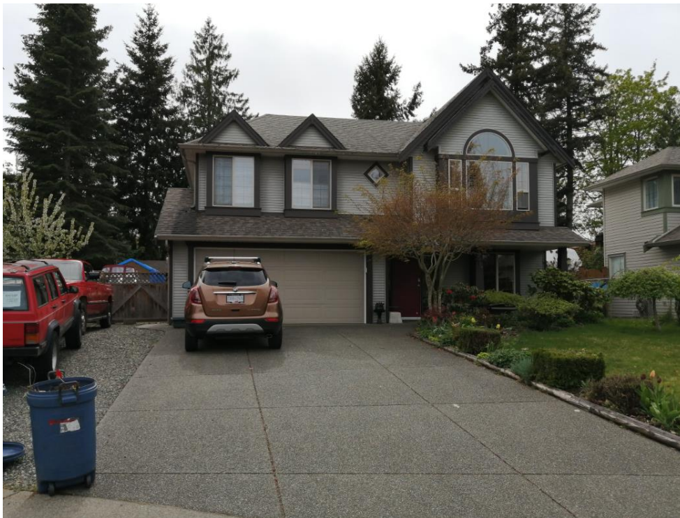
Figure 2. Existing home from Walbran Place.
